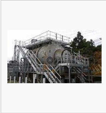
Front end of condenser unit
