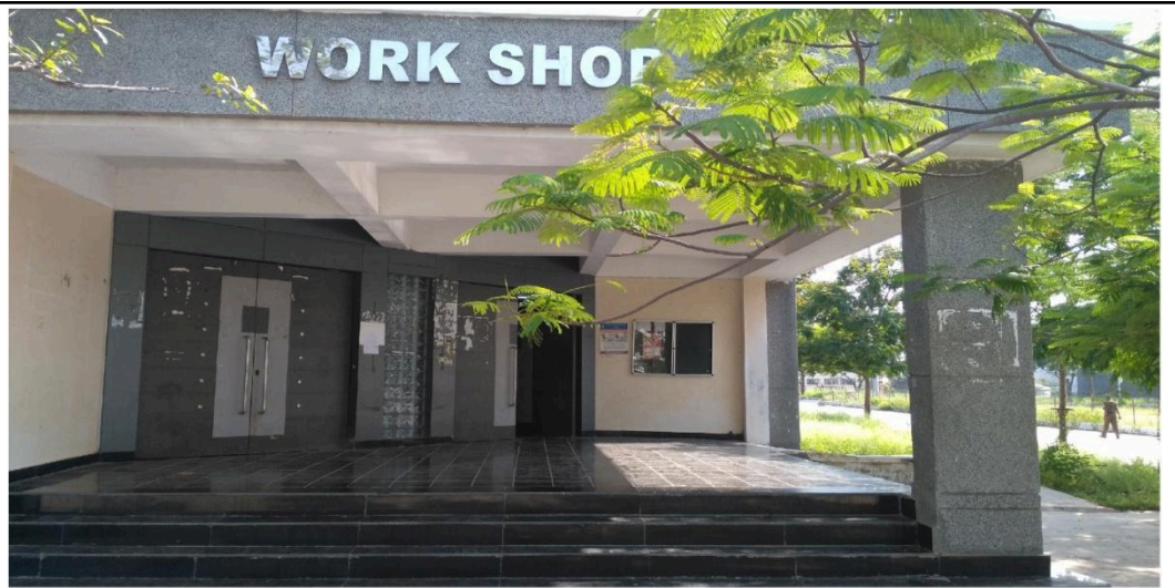
( Mechanical Workshop Building)
